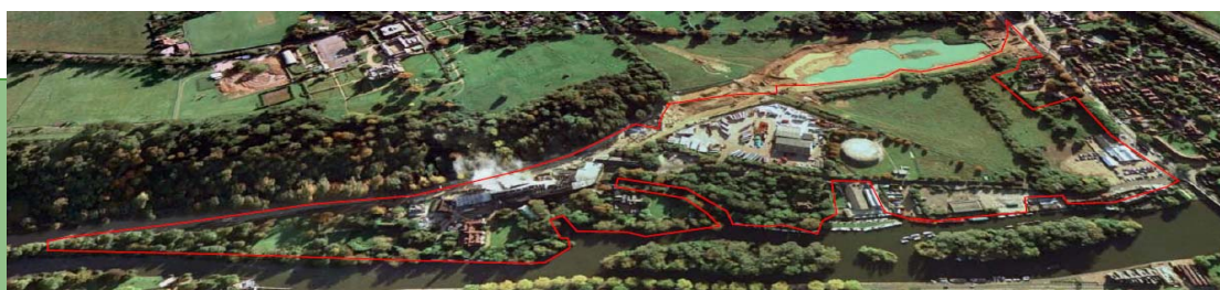
Photo: Mill Lane Strategic Site, Taplow
