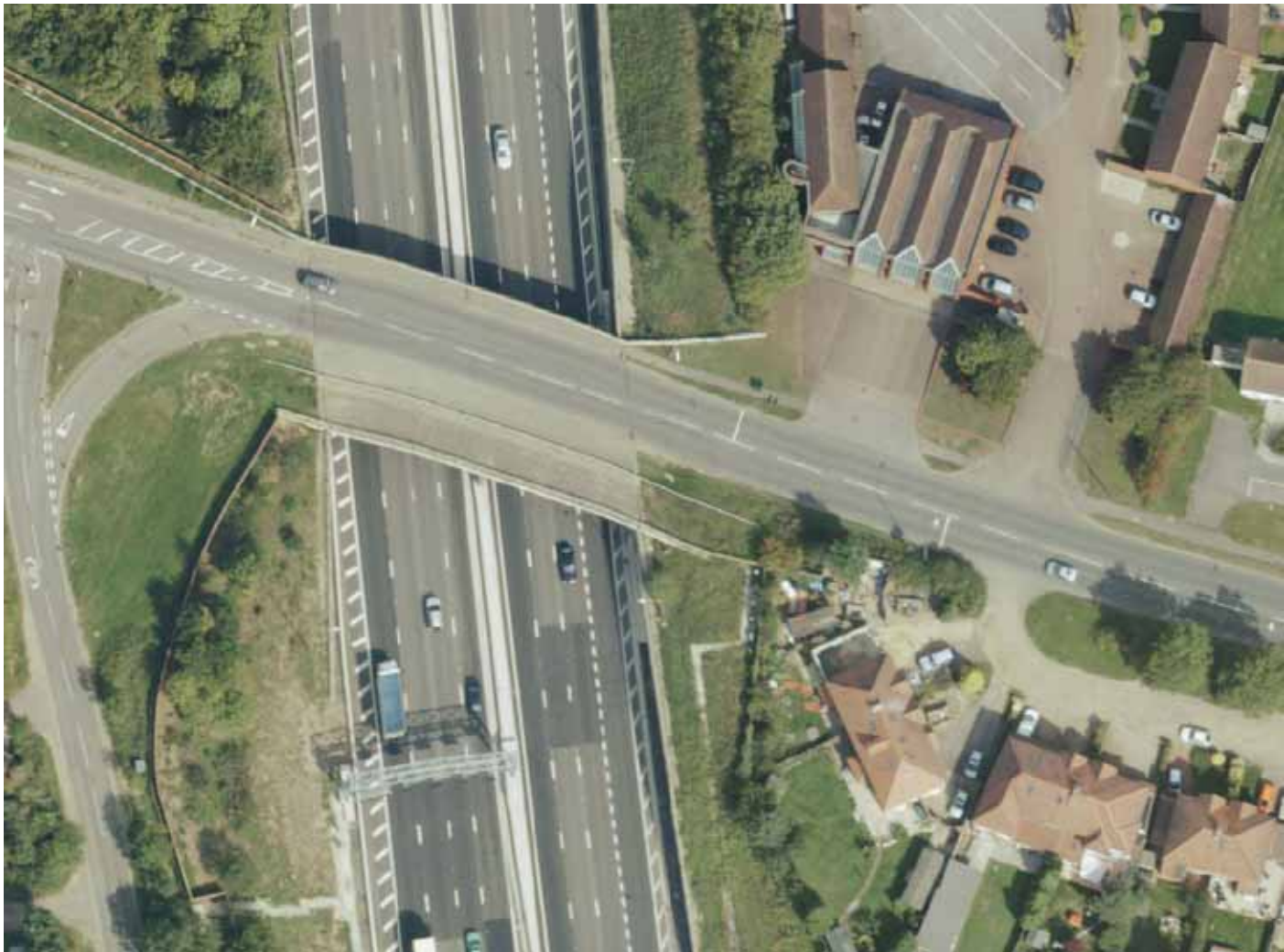
Figure 2.3: Aerial View of M25 after Completion of Widening Work.
