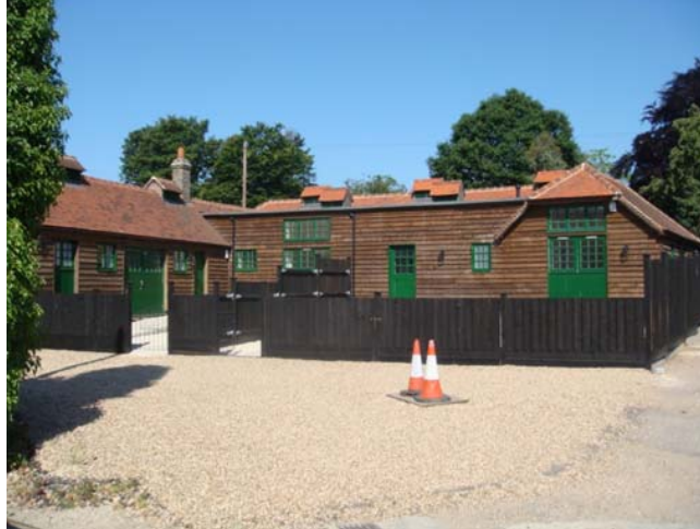
Britwell Road, Burnham (newly completed studios / workshops)
