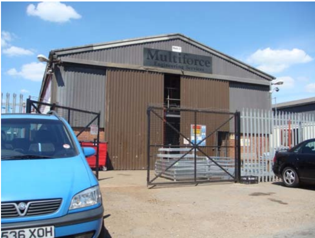
Court Lane, Iver (Multiforce Engineering Services)
